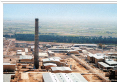
Uranium Conversion Facility (UCF), Isfahan. Here, uranium oxides are claimed to be produced as well as uranium hexafluoride and other uranium
