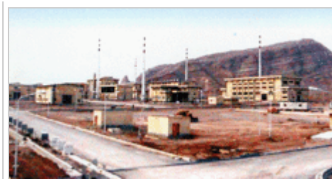
Zirconium Production Plant (ZPP), Isfahan, Iran. Here, special alloys are made that have direct applications in claddings for nuclear power plants. The ZPP plant is also capable of producing other special alloys for industrial purposes.
